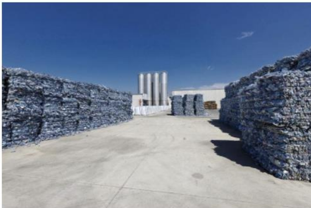
Aliplast industrial plant. (photo: Aliplast)
